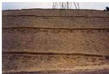
A sediment control log (SCL) captures eroded sediments and is considered a sediment control BMP.
