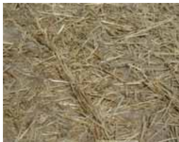
Seeding and mulching (SM) reduces erosion and is considered an erosion control.
