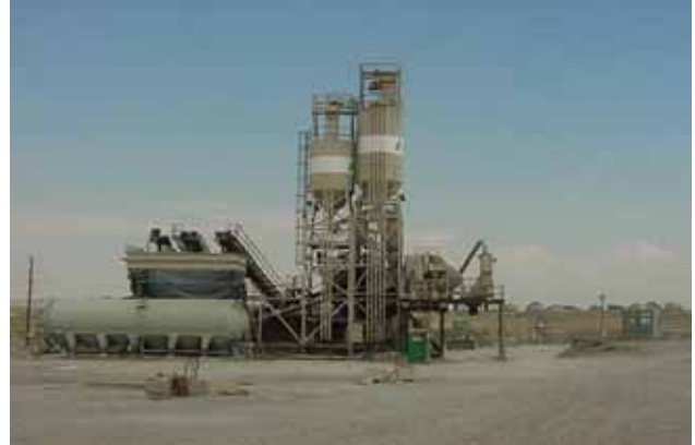
Temporary Batch Plants have specific GESC Plan requirements to reduce impacts to the environment.
