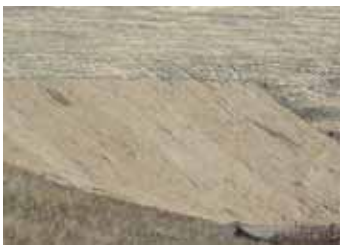
Erosion Control Blanket (ECB) shall be used on slopes greater than 4:1.
