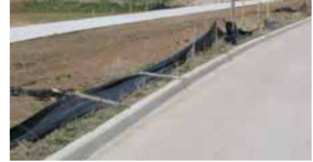
Silt Fence should be located far enough off streets to avoid damage from snow-plowing operations.
