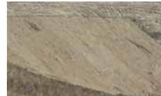
Erosion control blanket protecting a slope.
