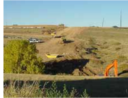
It is especially important to show Limits of Construction and erosion and sediment control BMPs for utility work outside the site.
