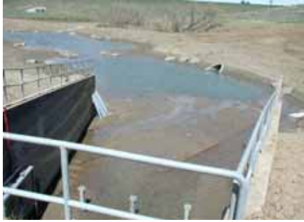
Sediment that accumulates in water quality ponds need to be cleaned-out periodically, requiring significant effort and cost.
