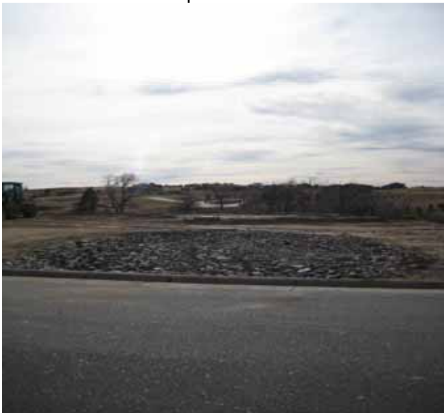
DO Properly installed vehicle tracking control.
