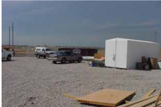
DO Properly installed stabilized staging area.
