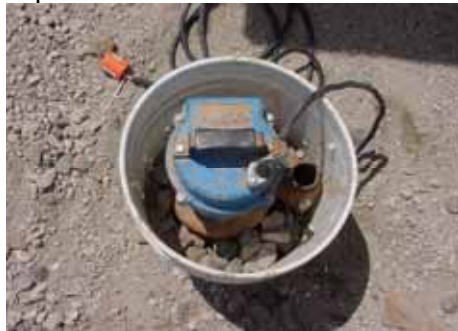
DO Sump pumps or suction lines can be contained within perforated 5-gallon buckets and surrounded with gravel to reduce the pumping of mud during dewatering operations.
