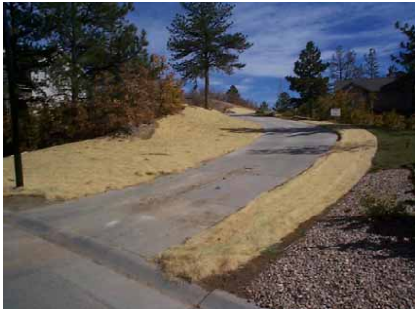
Erosion Control Blanket used to Stabilize Slopes
