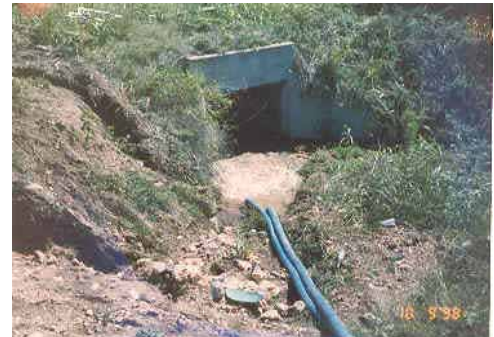
DON'T These discharge lines require a riprap pad and a settling trap.
