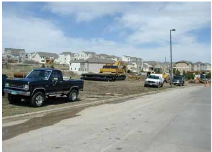
DO NOT Parking, staging, and storage are spread out all over this site, increasing disturbance and erosion.
