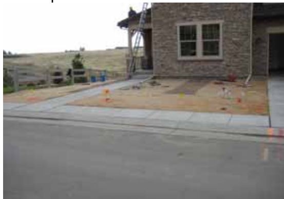
DO Erosion Control Blanket has been placed to control sediment movement on disturbed areas.
