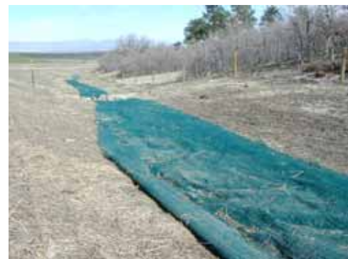
DON'T The edges of this erosion control blanket are not trenched in, allowing the blanket to become displaced.
