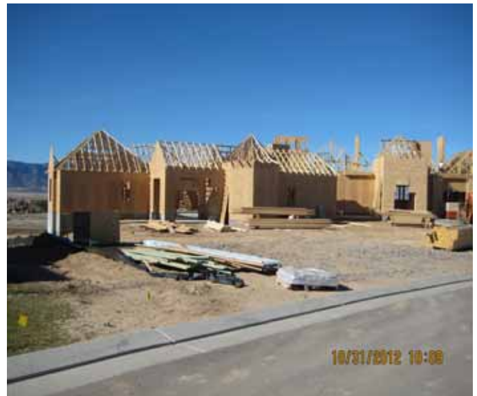
DONT The Vehicle Tracking Control Pad needs to be re-established on this site.
