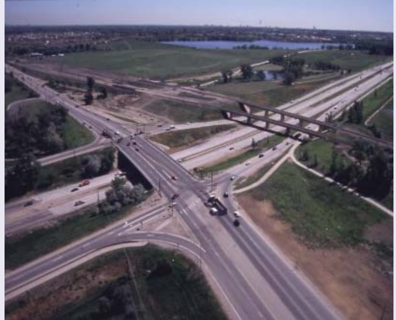
The above photo of the existing US 85/C-470 Interchange is taken looking northeast with C-470 running from left to right and US 85 running from top to bottom. It also shows the BNSF and Union Pacific railroads that both run adjacent to and east of US 85.
