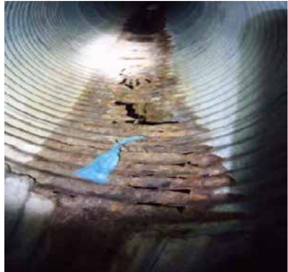
Corrugated Metal Drainage Pipe (CMP) – CMP has a design life of 30 + / - years, but many environmental factors can affect the actual length of the CMP life span. (Subsequent to the adoption of the Douglas County Storm Drainage Design & Technical Criteria Manual in 1986. CMP was no longer allowed for storm sewer installations).
