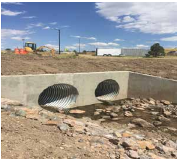
Culvert Repairs in Heritage Hills Park under construction (Pictured Left)
