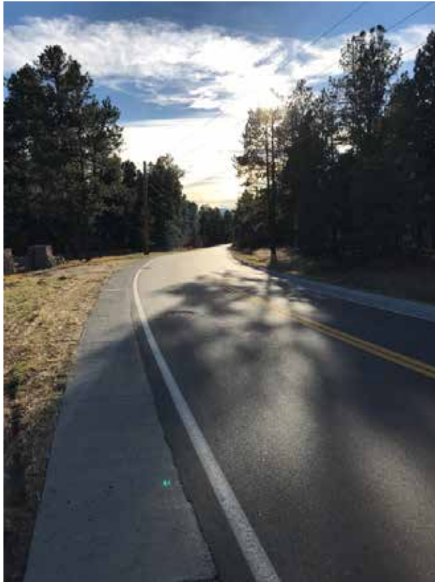
Happy Canyon Road – In 2017, the County rebuilt this rural collector roadway utilizing new centerline and edge-of-asphalt profiles in order to improve ride quality of the roadway and also provided a concrete apron to reduce erosion along the shoulder.
