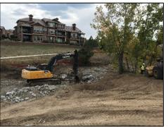
• **Sterling Ranch Filing #7-A and #5-C -** Three Sons Construction is installing storm sewer inlets in Filing #7-A, and Fiore is installing storm sewer in #5-C (DV#2023-410).
