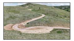
Construction on the south portion of Bluffs Regional Park trail was completed in May. DesignScapes Colorado was contracted to rebuild a section of Bluffs that was in need of improvements due to the safety concerns. The project included installing 800 tons of road base trail surface, retaining walls, cast in place concrete water bars, concrete pan culverts, and native grass seed.
