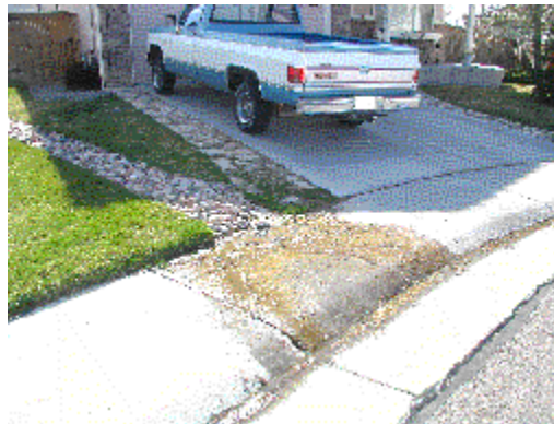
Photo 2 - Water flow and algae growth
