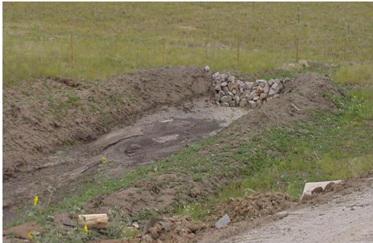
DO A properly installed sediment trap.
