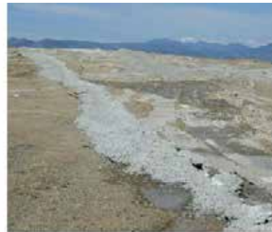
DO NOT Extensive wasting of concrete on the construction site requires additional effort to clean up and can impair subsequent revegetation operations.
