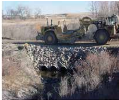
DO Properly installed temporary stream crossing.
