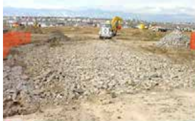
DO Properly installed vehicle tracking control.
