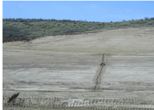
Surface roughening on this slope may have prevented this rill erosion.
