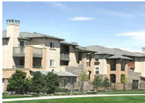
Multi-family projects require approval from both the Review Engineer and GESC Inspector.
