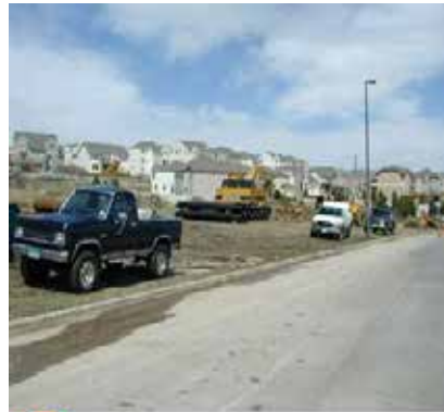
DON'T Parking, staging, and storage are spread out all over this site, increasing disturbance and erosion.
