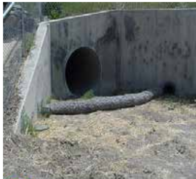
DO A properly installed reinforced rock berm for culvert protection.
