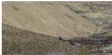
DO Ample erosion control blanket is used on this hill slope.
