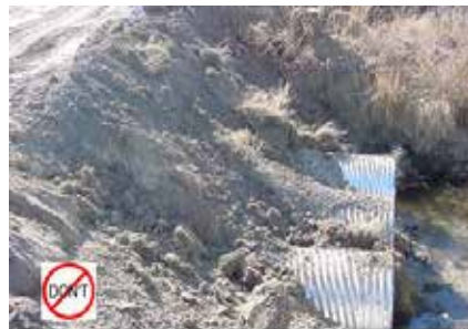
This temporary stream crossing is constructed of soil and is not acceptable.
