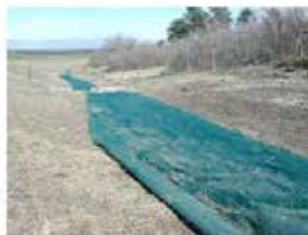
DONT The edges of this erosion control blanket are not trenched in, allowing the blanket to become displaced.
