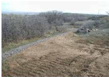
DO A reinforced rock berm may be used downgradient of disturbed areas in lieu of silt fence.
