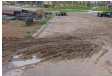
No vehicle tracking control means mud on streets and an immediate Stop Work Order.
