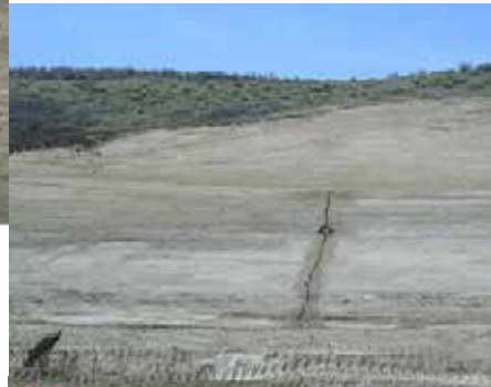
DO NOT Surface roughening on this slope may have prevented this rill erosion.
