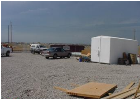
DO Properly installed stabilized staging area.
