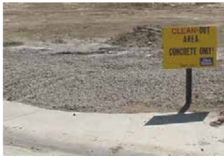
DO A properly installed concrete washout area with Vehicle Tracking Control.
