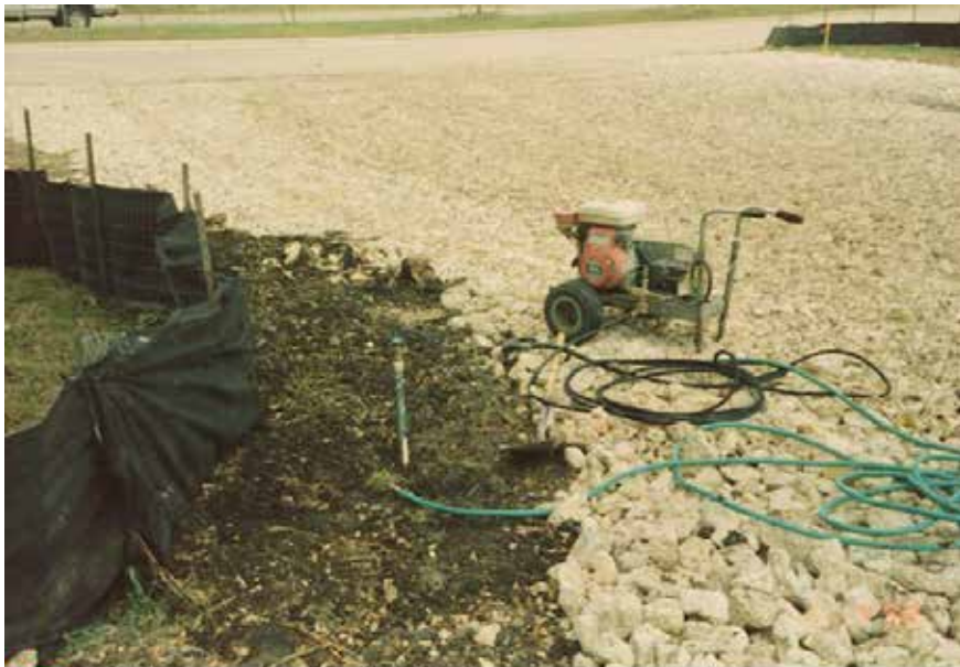
DO A high-pressure washer effectively cleans mud from wheels.
