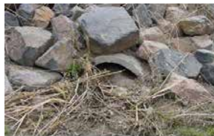
DO NOT Without a reinforced rock berm for culvert protection, culverts fill with sediment.
