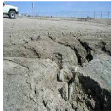
DO NOT Lack of a diversion ditch at the top of this slope to divert upstream runoff has led to severe rill and gully erosion.
