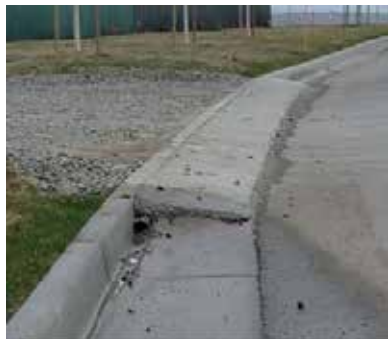
Curb ramps of earth, concrete, or lumber are not permitted in the curb section.
