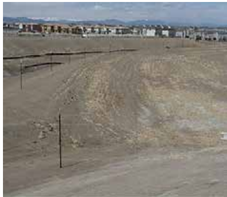
DO This diversion ditch provides protection for an adjacent drainage way.
