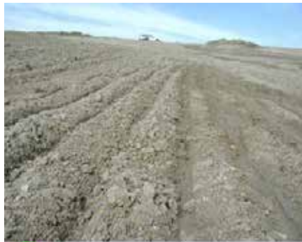
DO Properly executed surfacing roughening.
