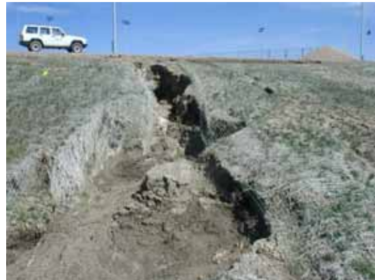
Control of construction site erosion in Douglas County is mandated by Federal and State law.
