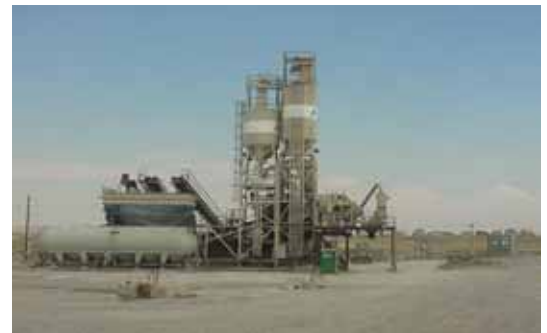
A Temporary Batch Plant requires its own GESC Permit.
