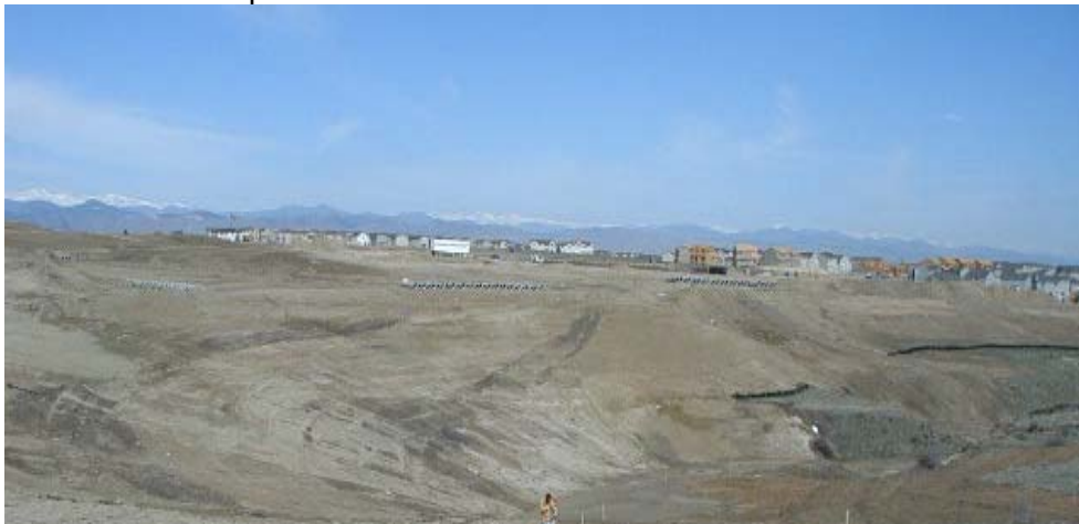
Large areas of disturbance create huge potential for erosion and sedimentation; limiting the area of disturbance substantially reduces the problem.
