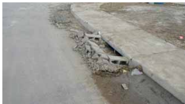
DON'T Tubular markers were not placed in front of this inlet protection installation, making it more susceptible to damage from snowplows and other vehicles. This installation is in need of immediate repair.
