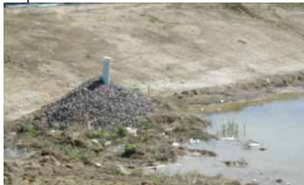
DO Properly installed outlet pipe and gravel pack.
