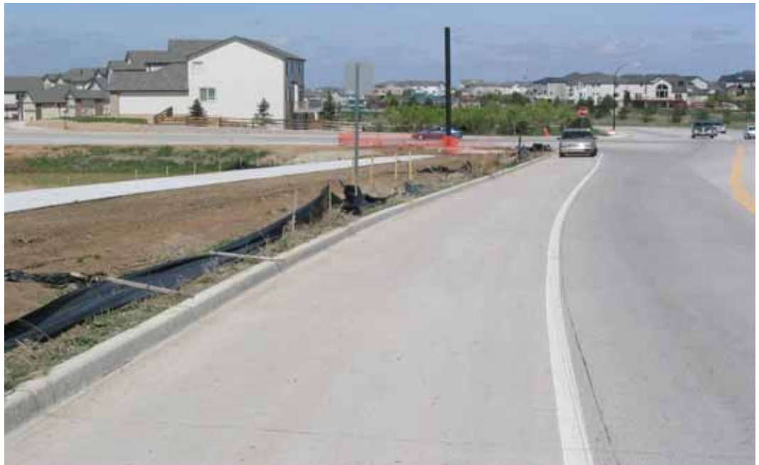
Maintenance procedures are not being followed on this site which may lead to additional costs from reinspection fees, sediment clean up and possible work stoppages.
