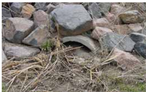
DON'T Without a reinforced rock berm for culvert protection, culverts fill with sediment.
