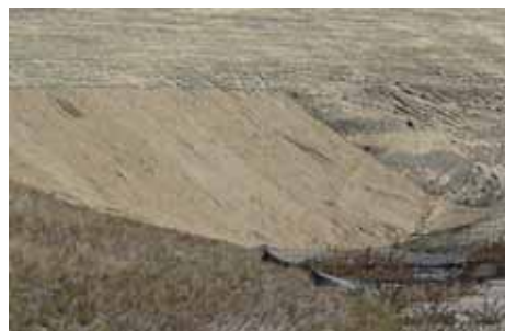
DO Ample erosion control blanket is used on this hill slope.
