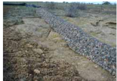
DO Reinforced rock berms are especially useful over bedrock outcroppings or pavement where silt fence and sediment control logs cannot be installed.
