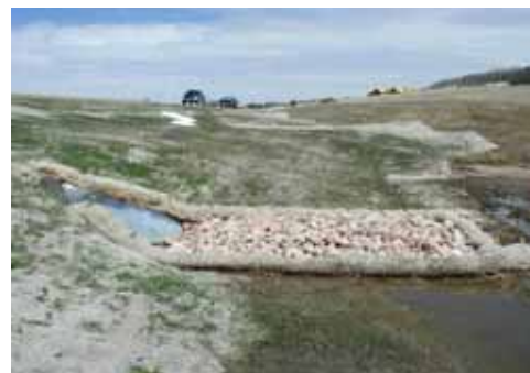
DON'T Although some sediment trapping would occur with this alternate arrangement, the standard detail shall be utilized.
