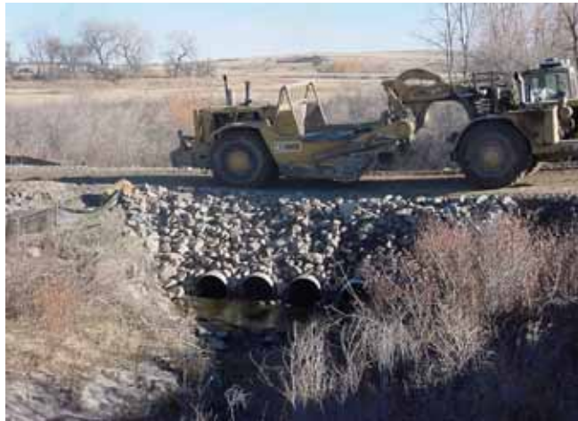
DO Properly installed temporary stream crossing.
