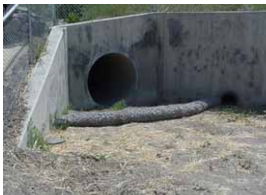
DO A properly installed reinforced rock berm for culvert protection.
