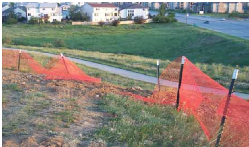
DON'T This construction fence is in need of repair. Inspections shall be made daily and downed sections repaired immediately.
