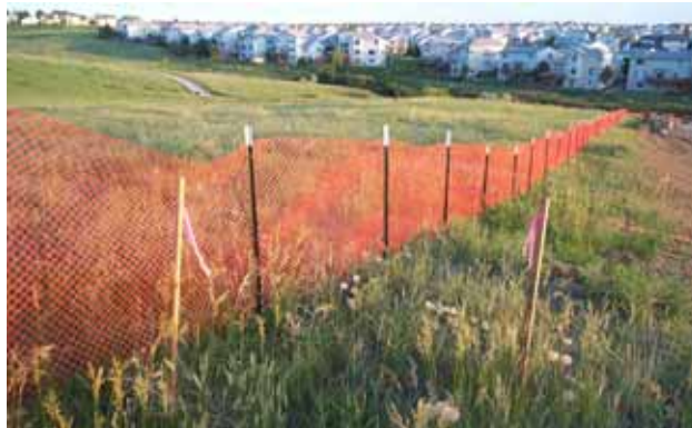
DO Use construction fence to restrict access to site and demark limits of disturbance.
