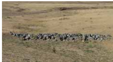
DO Properly installed check dam.
