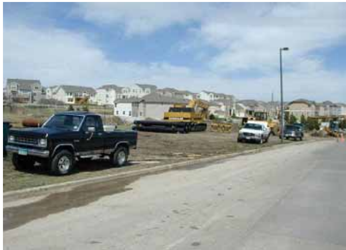
DON'T Parking, staging, and storage are spread out all over this site, increasing disturbance and erosion.
