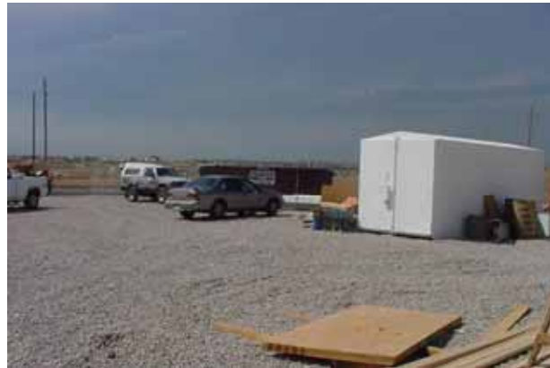
DO Properly installed stabilized staging area.
