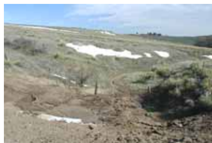
DO NOT This disturbed drainageway was not protected by a check dam at the downstream site perimeter, allowing sediment to be conveyed off site.
