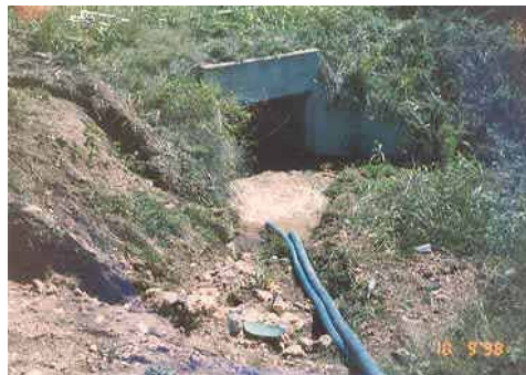
DON'T These discharge lines require a riprap pad and a settling trap.
