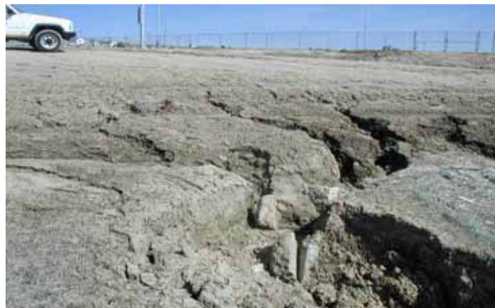
DO NOT Lack of a diversion ditch at the top of this slope to divert upstream runoff has led to severe rill and gully erosion.
