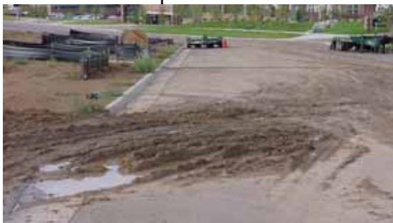
DON'T No vehicle tracking control means mud on streets and an immediate Stop Work Order.
