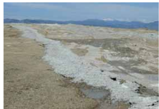
Extensive wasting of concrete on the construction site requires additional effort to clean up and can impair subsequent revegetation operations.
