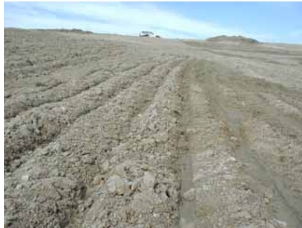
DO Properly executed surfacing roughening.
