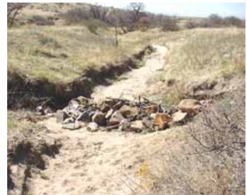
DO NOT This check dam was not keyed in adequately to the channel bank, leading to its failure.
