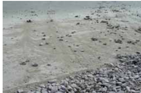
DON'T Use of low density rock such as Rhyolite is not permitted since it does not stay in place and can get tracked onto paved streets.
