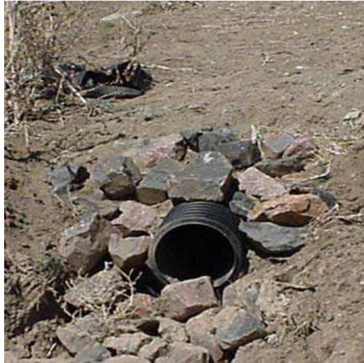
DO Properly installed temporary slope drain pipe alternative.
