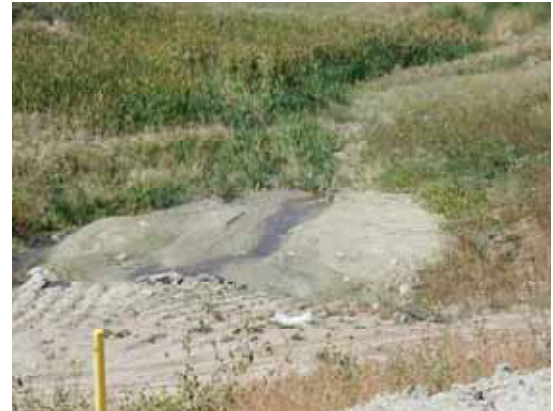
Lack of construction fence to define limits of construction can lead to unnecessary disturbance in drainageways.
