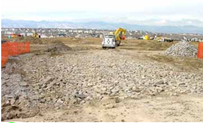
DO Properly installed vehicle tracking control.
