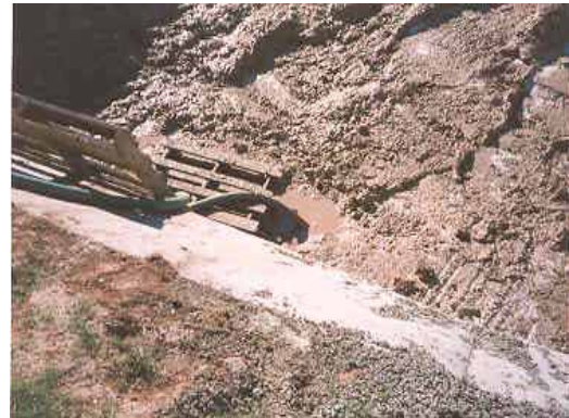
DON'T This suction line is not contained in gravel and is pumping excessive amounts of sediment.
