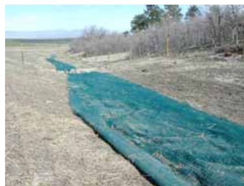
DON'T The edges of this erosion control blanket are not trenched in, allowing the blanket to become displaced. Blanket shall be 100% natural and biodegradable.
