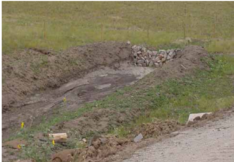
DO A properly installed sediment trap.
