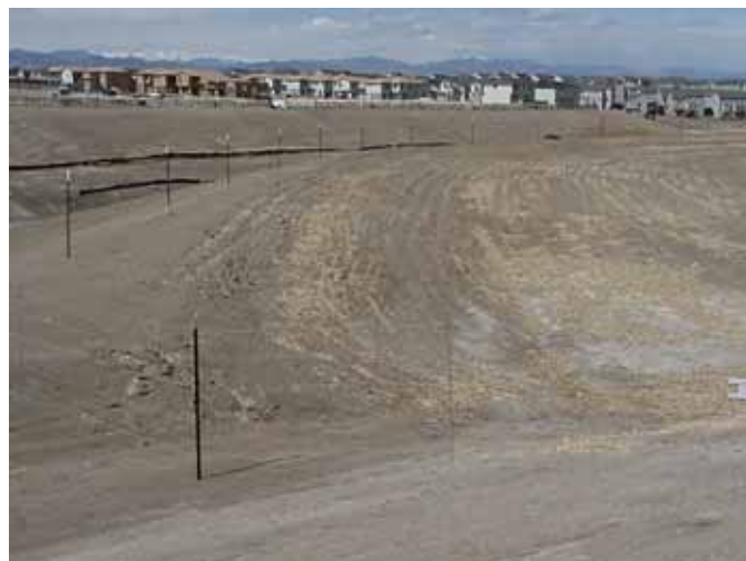
DO This diversion ditch provides protection for an adjacent drainageway.
