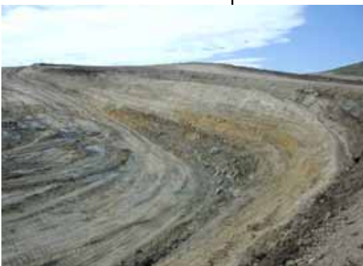
Excavation and fill shall take place under controlled conditions in accordance with recommendations of a licensed Geotechnical Engineer.
