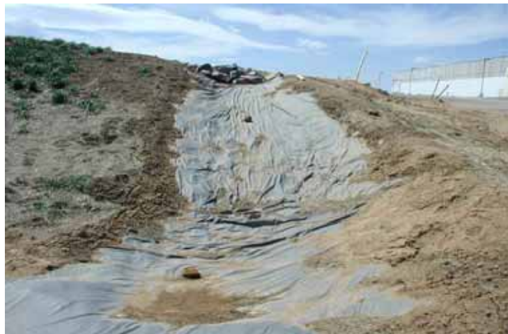
DO This plastic lined temporary slope drain allows runoff to be conveyed down a slope without causing rill and gully erosion.
