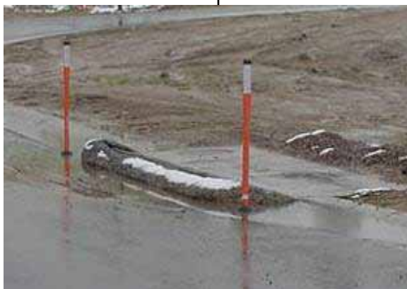
DO Properly installed inlet protection for curb-inlets in a sump condition.
