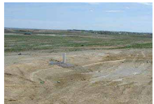
DON'T The sediment basin above is improperly installed due to: • Lack of an armored spillway. • Pipe perforations set above the spillway crest elevation.
