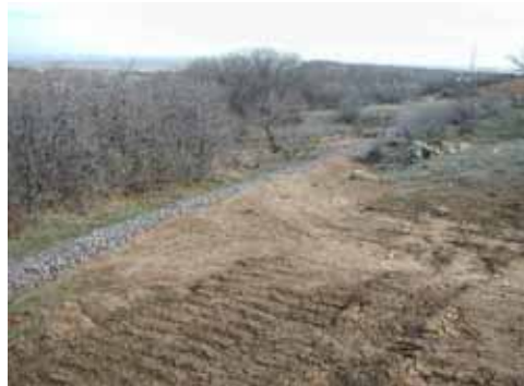
DO A reinforced rock berm may be used downgradient of disturbed areas in lieu of silt fence.
