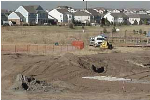
Construction fence helps a GESC Manager restrict operations to the defined limits of construction.
