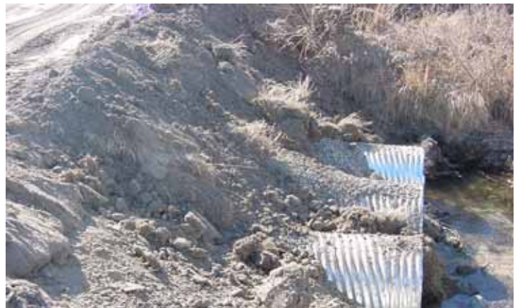
DON'T This temporary stream crossing is constructed of soil and is not acceptable.
