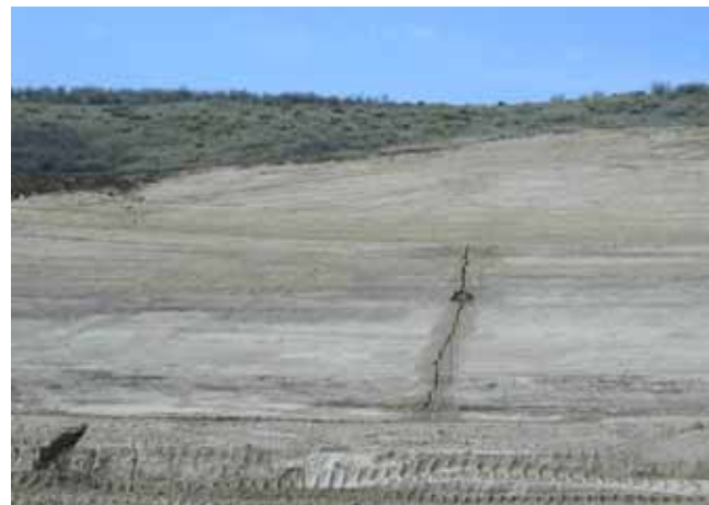
DO NOT Surface roughening on this slope may have prevented this rill erosion.
