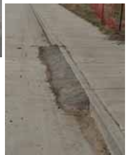
DON'T Curb ramps of earth, concrete or lumber are not permitted in the curb section.
