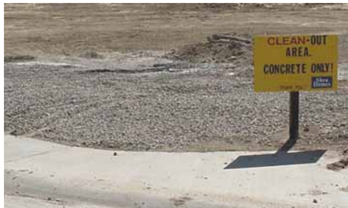
A properly installed concrete washout area with Vehicle Tracking Control.
