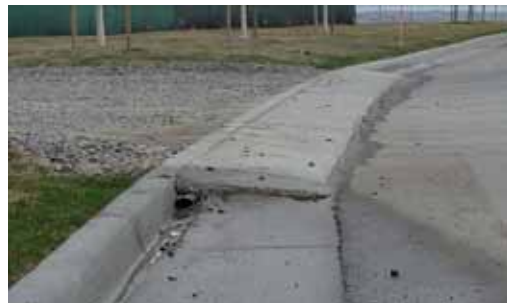
DON'T Curb ramps of earth, concrete or lumber are not permitted in the curb section.
