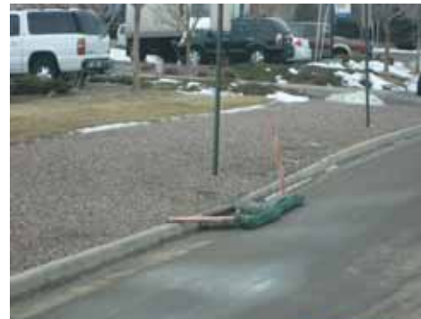
Fabric filter bags are not a Douglas County approved inlet protection BMP. See the Small Utility GESC Plan Standard Notes and Details (Appendix B) for the approved inlet protection details.
