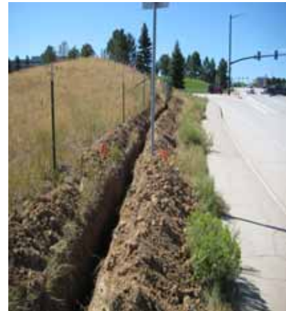
Failure to install BMPs prior to the start of a utility project shall result in the issuance of a Stop Work Order.
