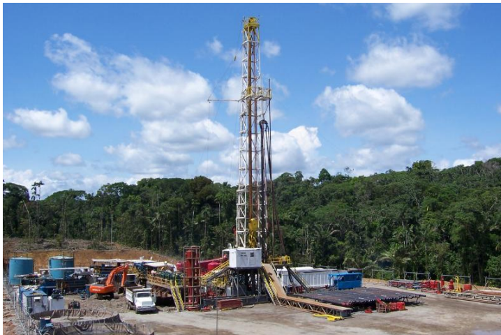
Nabors 818 drilling rig and pad site Source: Harris Drillina, LLC, oil & gas development consultants
