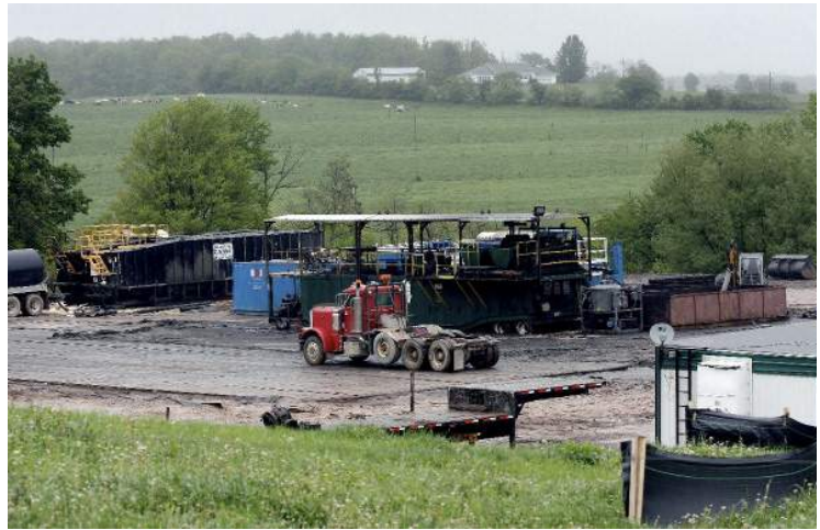
A natural gas well pad under construction in Springfield Township, PA Source: Democrat and Chronicle Newspaper, Rochester, NY, June 2011
