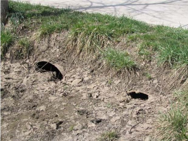
Another important part of maintaining a roadways drainage system is keeping the culverts and inlets clear of debris and sediment. Much like the roadside ditch, the culverts and inlets were designed to carry a certain amount of stormwater flow, and as the capacity of the culverts/inlets are reduced by clogging with debris and sediment, so is the ability for the overall stormwater system to adequately convey flows away from the road.
