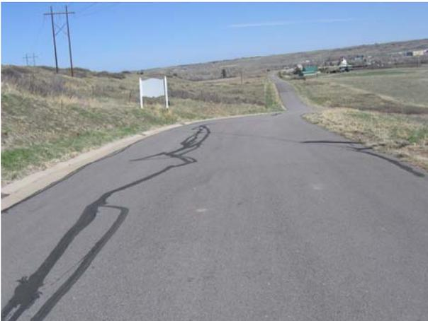
Curb and gutter is identified in Douglas County criteria as one alternative for roadside drainage conveyance in the rural areas. While many people don't view curb and gutter as looking very "rural", it can serve an important purpose in roadway design in the rural parts of the County.
