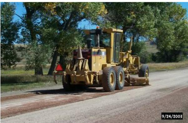
While maintaining the proper crown on a paved roadway takes little to no effort, the same cannot be said about a gravel road. Preserving the proper crown on a gravel road can involve infrequent maintenance (once every two years) or very frequent maintenance (numerous times a year), depending on the amount and type of traffic using the gravel road, the original design and construction of the road and other factors, such as weather. A motor grader operator can
